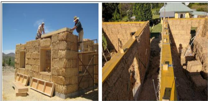
Figure 1: Straw- load-bearing and the in filling. Source: [12].
