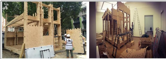
Figure 16: Made entirely from digitally fabricated components, a CNC milling machine laser-cuts the necessary pieces out of fiberboard, which can be assembled without the need for any additional materials like screws and fixtures. Source: [10].
