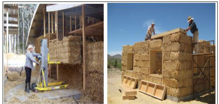
Figure 2: Straw - The post and beam system. Source: [12].
