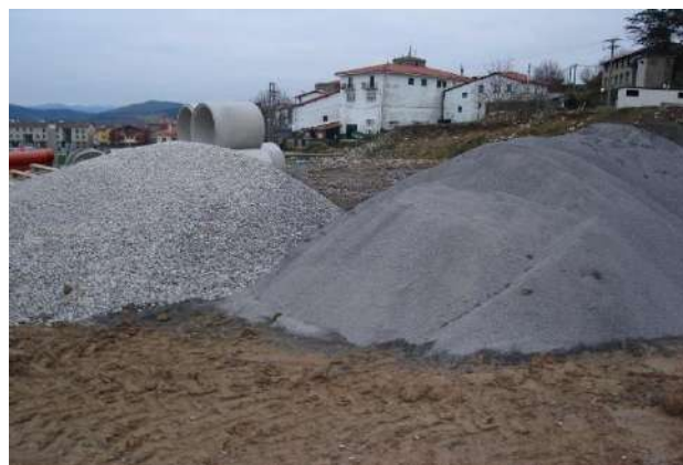
Figure 5 - Aggregate for the preparation of mortar. Source: Authors, (2019).
