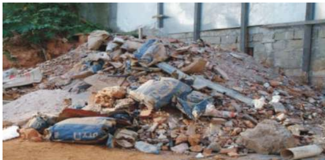
Figure 2 - Incorrect Waste Disposal. Source: [15].
